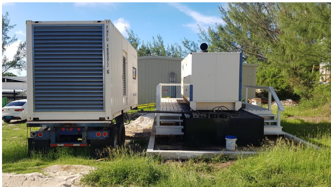
Figure 2.8 Diesel backup power generator
