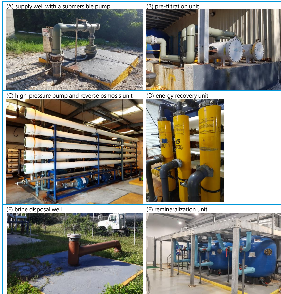
Figure 2.3 Facilities in a typical SWRO plant
